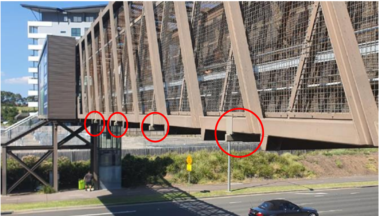
FIGURE 6: OUTRIGGERS SUPPORTING THE BOTTOM OF THE EASTERN AND WESTERN SIGNBOARDS
