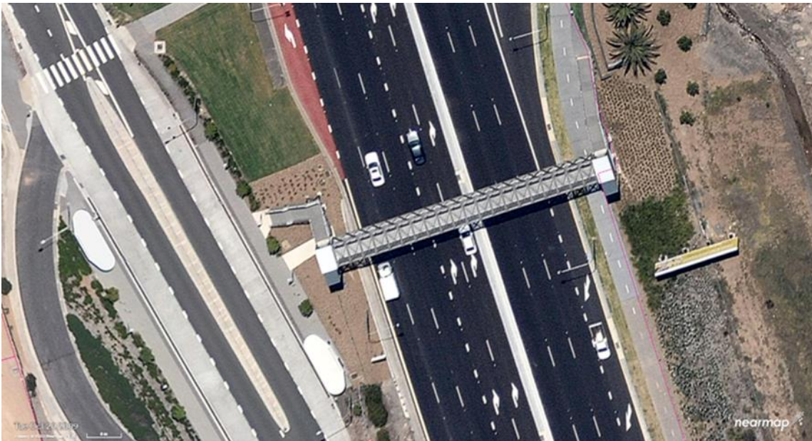
FIGURE 1: PEDESTRIAN BRIDGE ON 20 OCT 2009 (SOURCE: NEARMAP)
