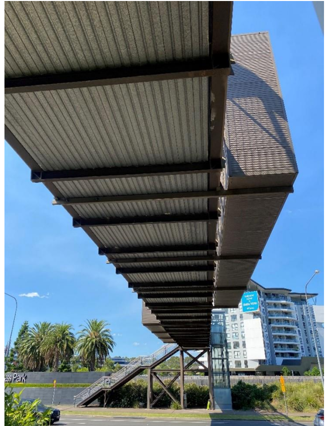
FIGURE 5: OUTRIGGERS SUPPORTING THE BOTTOM OF THE EASTERN AND WESTERN SIGNBOARDS
