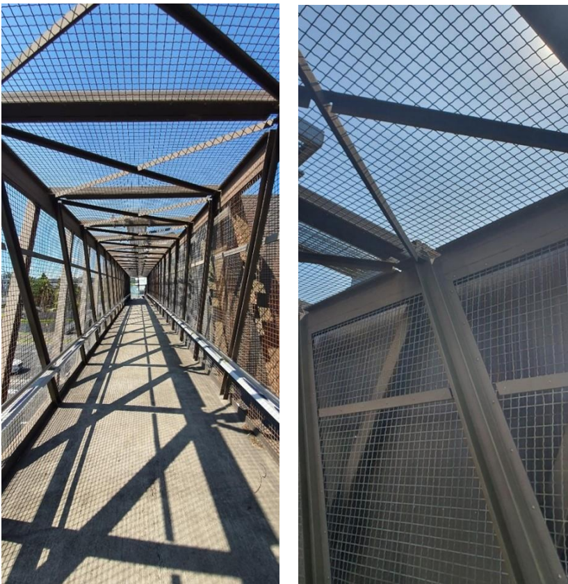
FIGURE 8: DECK OF BRIDGE AND BRIDGE FRAMING AT THE BACK OF THE SIGNBOARD
