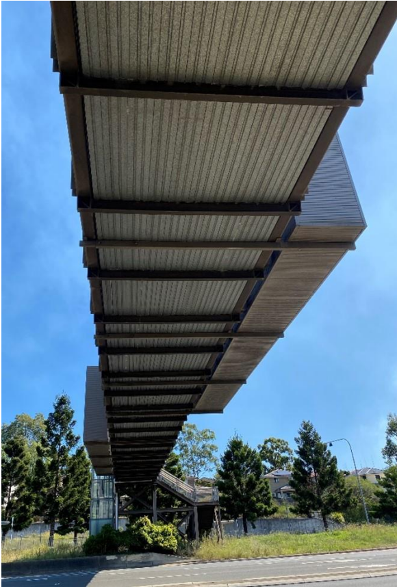
FIGURE 5: OUTRIGGERS SUPPORTING THE BOTTOM OF THE EASTERN AND WESTERN SIGNBOARDS
